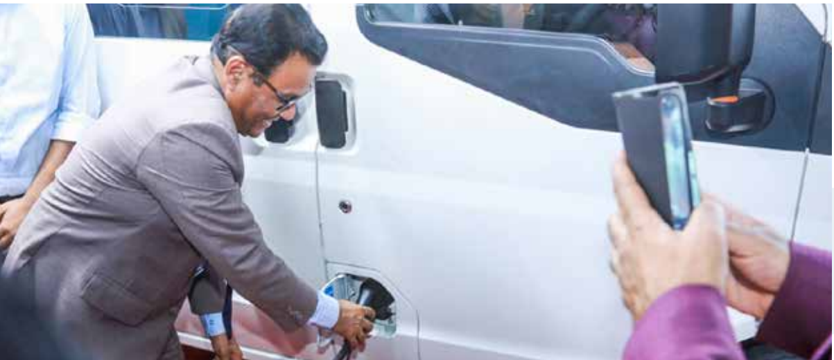
DESCO inaugurated Electric Vehicle Charging point at Matikata in Dhaka
