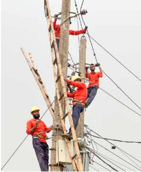
Cable Maintenance Works of DESCO at Vhatara Area
