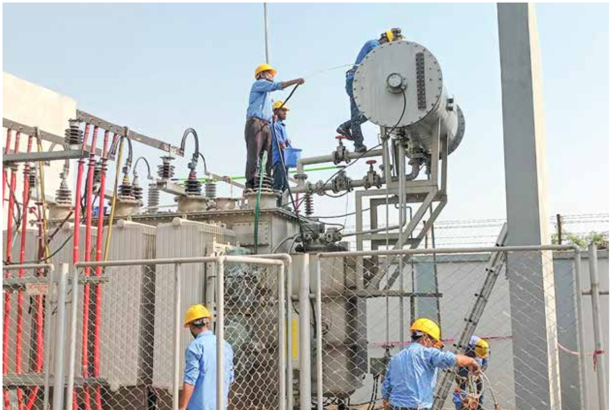
Periodical Substation Maintenance works at Baridhara Substation
