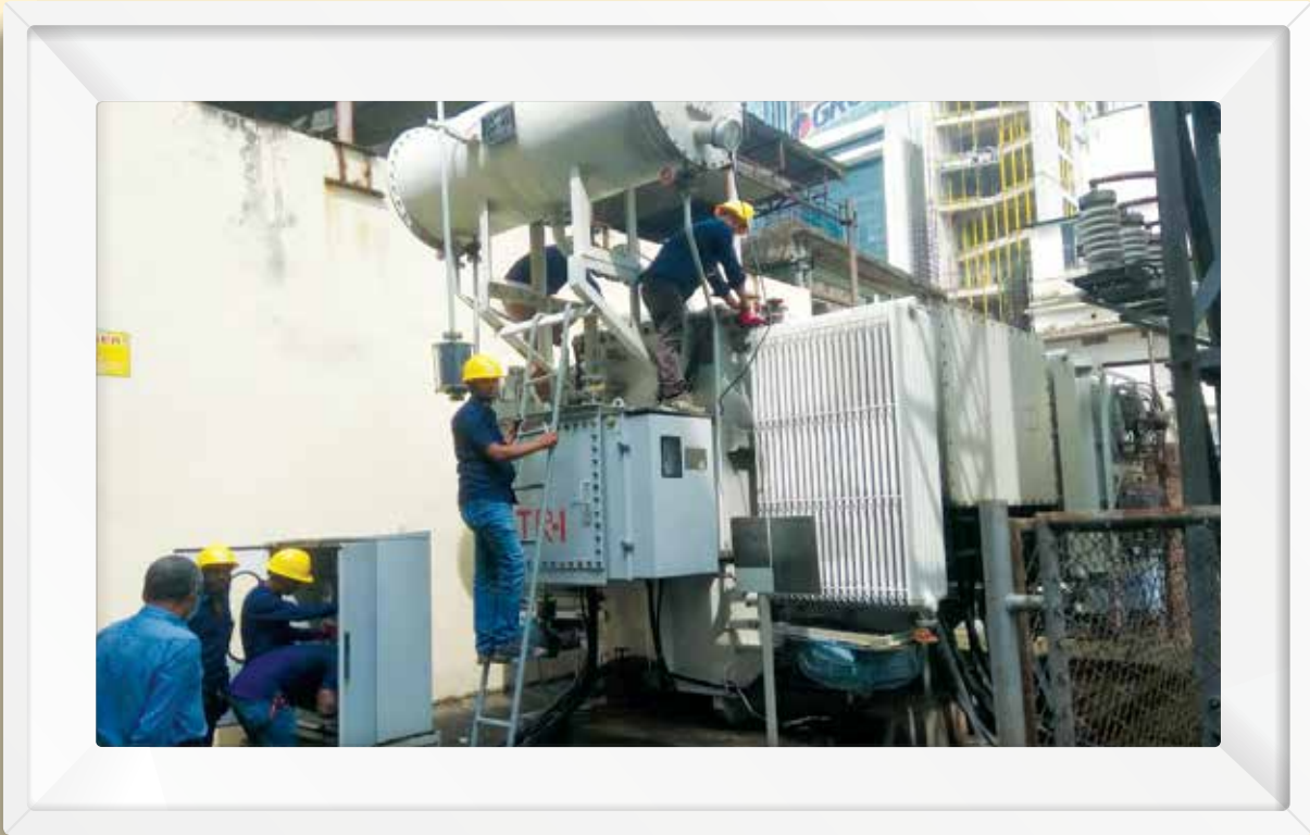
Transformer Maintenance Works
