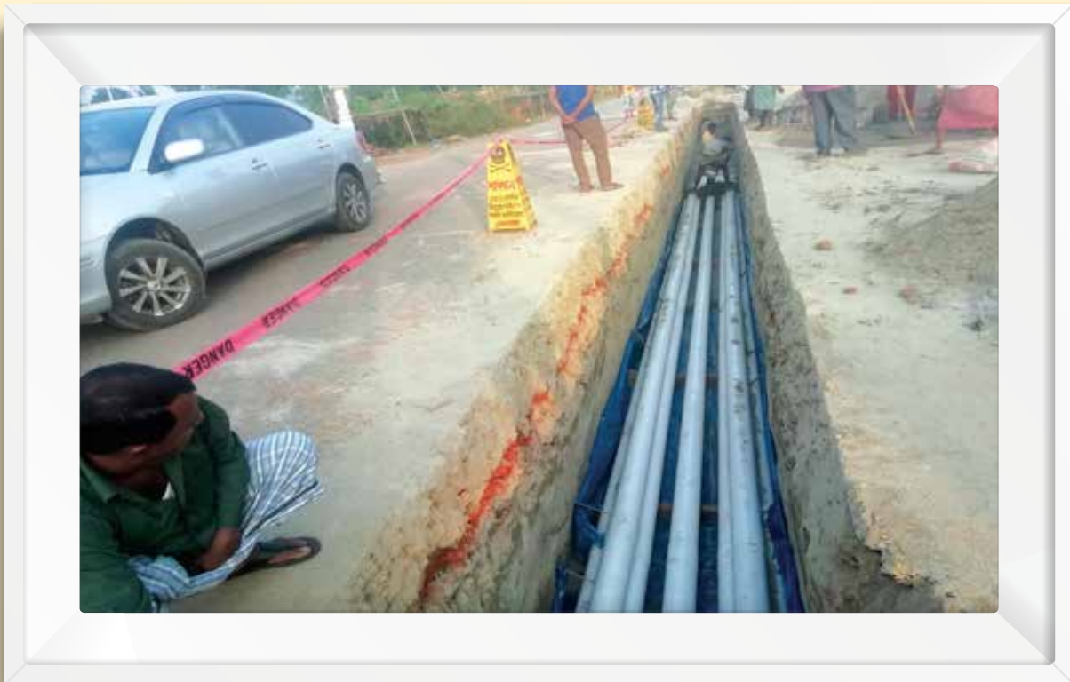
Electric Cable Underlying Works in DESCO Area
