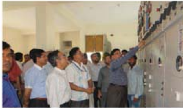
Visit of Sub-stations
