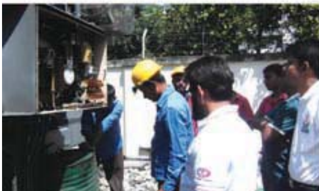
Schedule Maintenance of Sub-stations
