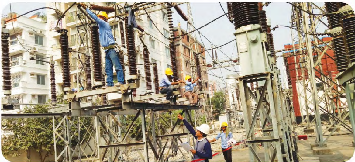
Outdoor Maintenance Work
