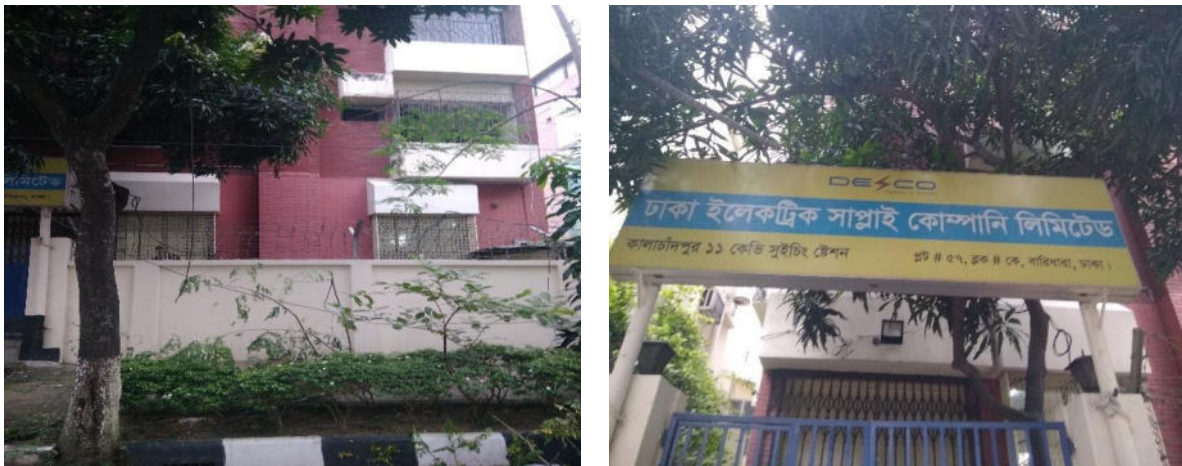
Figure 4.11: 11 kV Switching Station at Proposed Project Location
