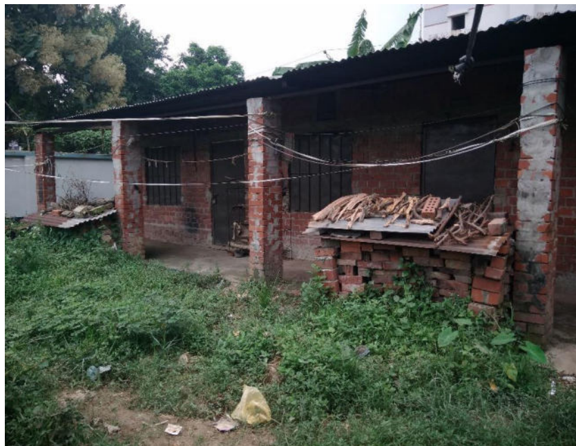
Figure 4.15: Workers Shed in Proposed Substation Area
