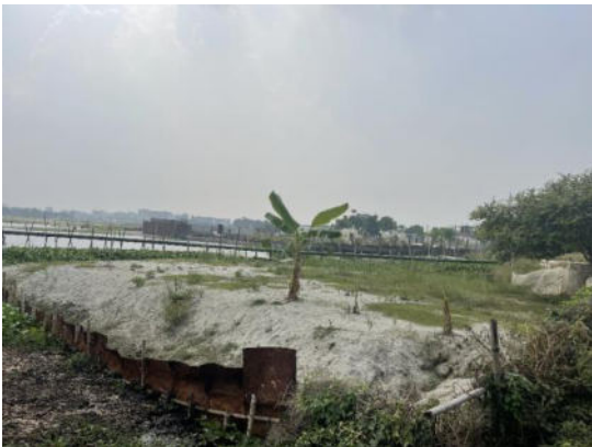
Figure 4.20: Sand Filling
