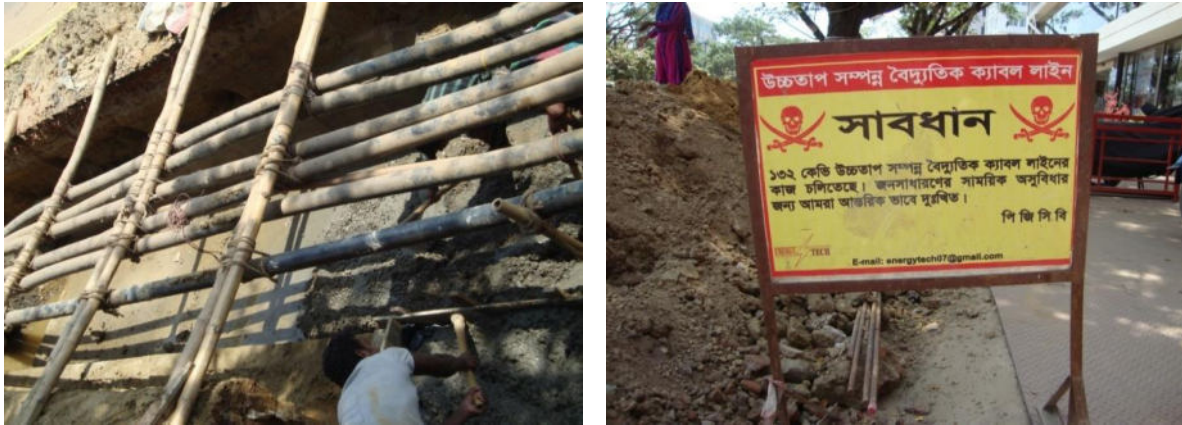
Figure 4.22: 132 kV Cable Trenching Work
