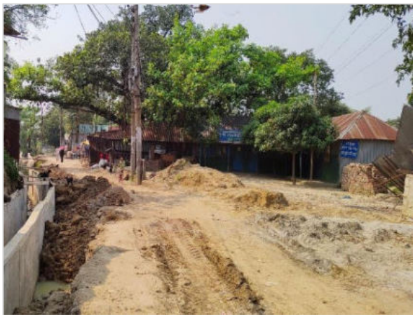
Approach Road of Proposed Tongi Substation (post-photo construction now complete)
