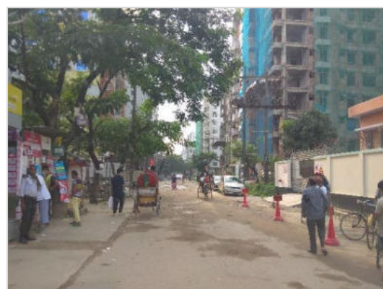
Road side infrastructure at Bashundhara Area
