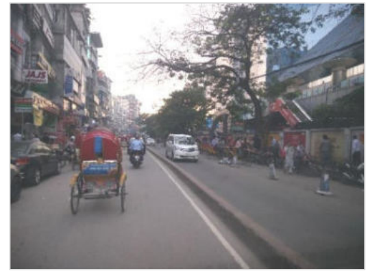
Road side infrastructure at Bashundhara area
