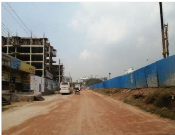
Cable Route at Kalshi Point
