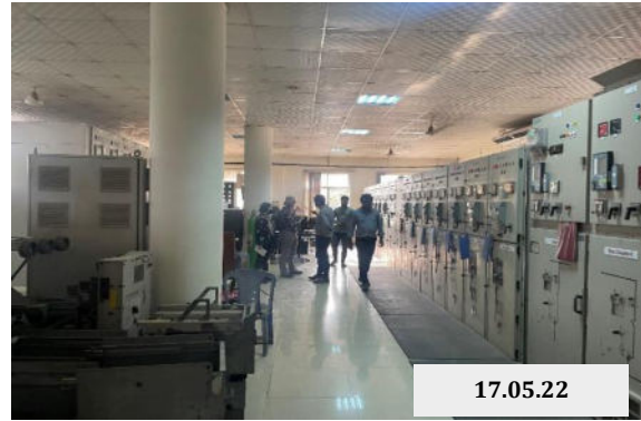
Consultation by ADB TA consultants at Kalachndpur SS site
