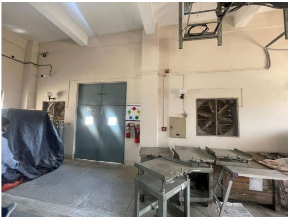
Photo-20: Exhaust fan for ventilation at Uttara SS and same was found in all other SS
