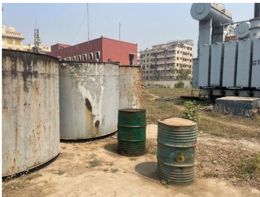
Photo-4: Damaged transformers and waste oil barrels store on open ground at Uttara 132/33/11 kV grid SS site.
