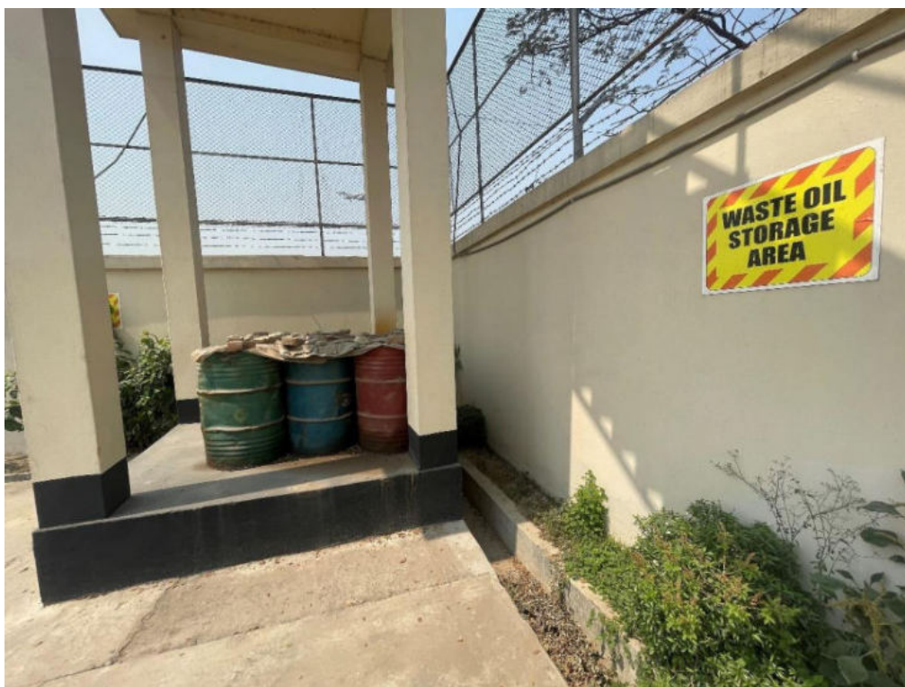
Photo-3 Waste oil stored without secondary containment at Uttara 132/33/11 kV grid SS site.
