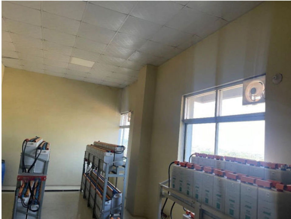
Photo-19: Exhaust fan for ventilation in battery room
