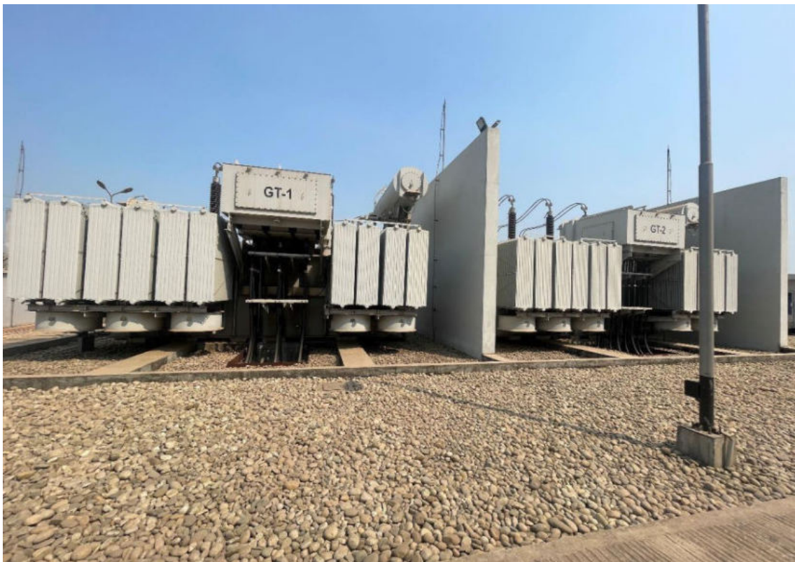
Photo-6: Set up transformer at Purbachal S2 132/33/11 kV grid SS site
